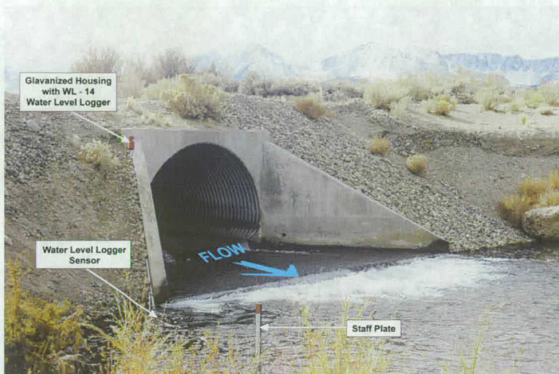
Figure 7. Rush Creek gaging station installation at the County Road culvert.
