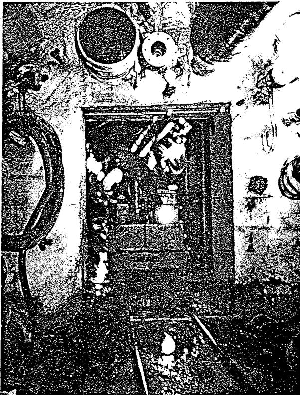
(Top) Section of completed concrete lined tunnel in Heading No. 4, looking west. (Above, left) Reinforced concrete bulkhead, fitted with steel door, installed in Heading No. 2 for use in emergencies. (Right) Water flow of 1500 gallons per minute pouring into Heading No. 3 of the 11-mile tunnel.
