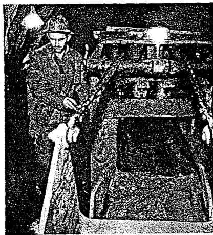
*MonoCraters Tunnel Project scenes and equipment: (Above) Drill carriage with machines in operation at tunnel face. (Left) Mucking machine removing material from tunnel face. (Below) One of two tunnel ventilating blowers equipped with 150 horsepower auxiliary gasoline engine driven motor, ready for shipment to Project. (Right top) Ship and cage, designed and built in Department shops. (Right bottom) one of twelve special pumps used in tunnel.*
