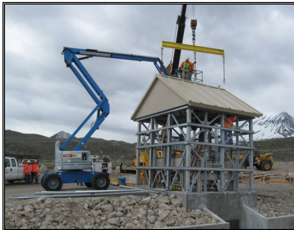
Photo 2: Roof installation
