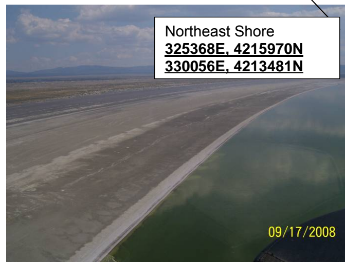
Figure 13. Northeast Shore AreaT
