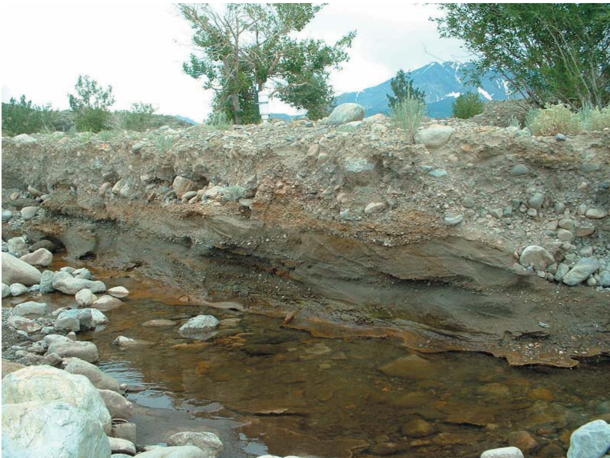
Figure 10. Cut-bank at Rush Creek 3D side-channel eroded during the June 2004 SRF releases, exposing underlying sediments and stratigraphy.
