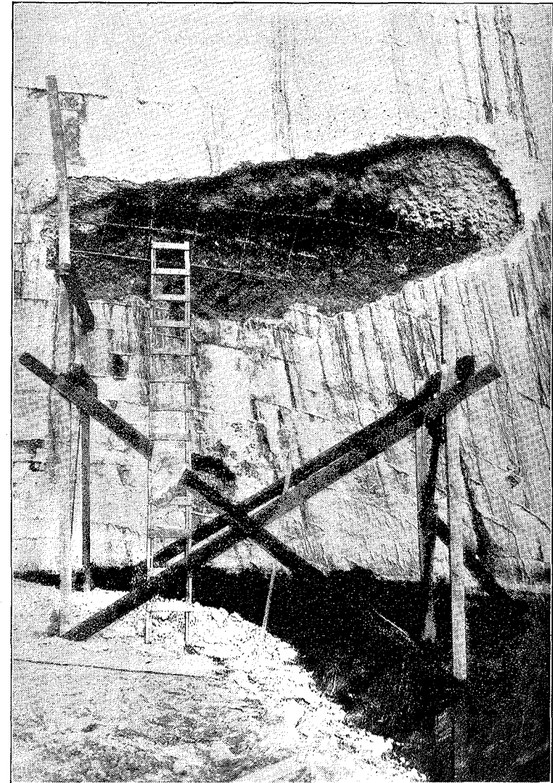
FIG. 7.—EXPLORATION IN REAR FACE OF GEM DAM EXPOSING REINFORCEMENT.
