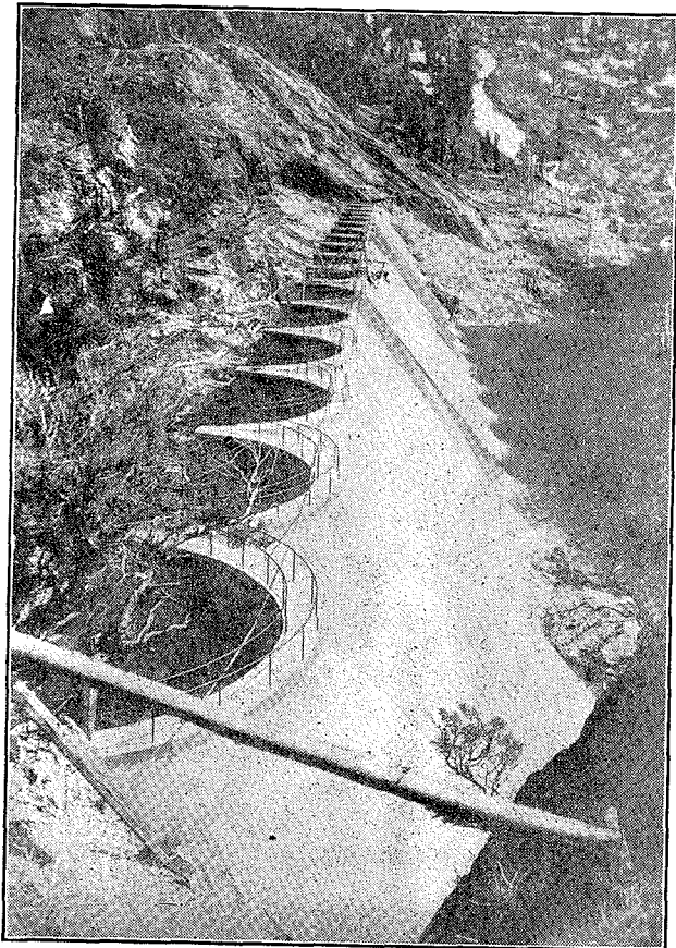
FIG. 4.—GENERAL VIEW OF GEM DAM.
